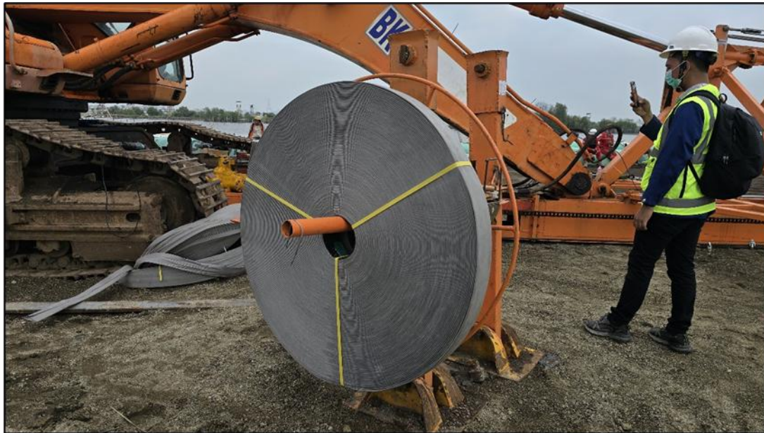
Figure 2. Prefabricated Vertical Drain (PVD)
